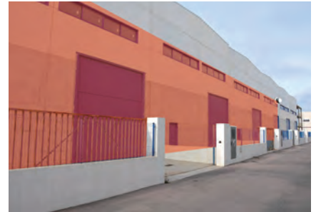
Wall protection (outdoor) at Warehouse
